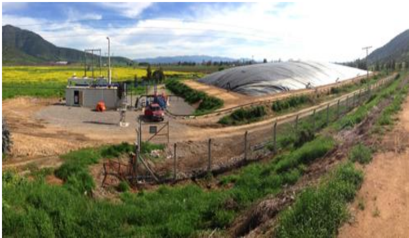
FIGURE 1: SANTA IRENE POWER PLANT
